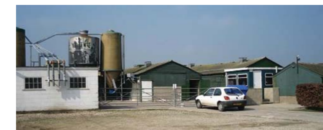
Entrance to unit showing single staff entrance, changing and showering unit
